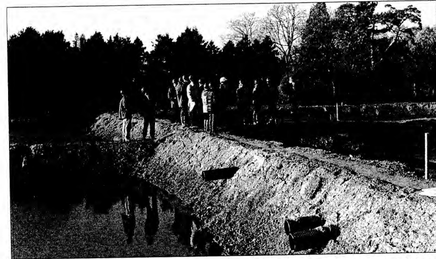
Removal of sediment to be deposited in these lagoons from Barton Broad, will recreate sufficient depth for recreation and navigation. Subsequent biomanipulation should re-establish clear water and conservation value.
