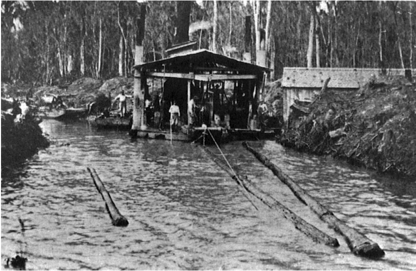
FIGURE 4.15 A two-drum pull boat working in a canal that was cut into a cypress swamp in Louisiana (date unknown). (From Williams 1989.)
