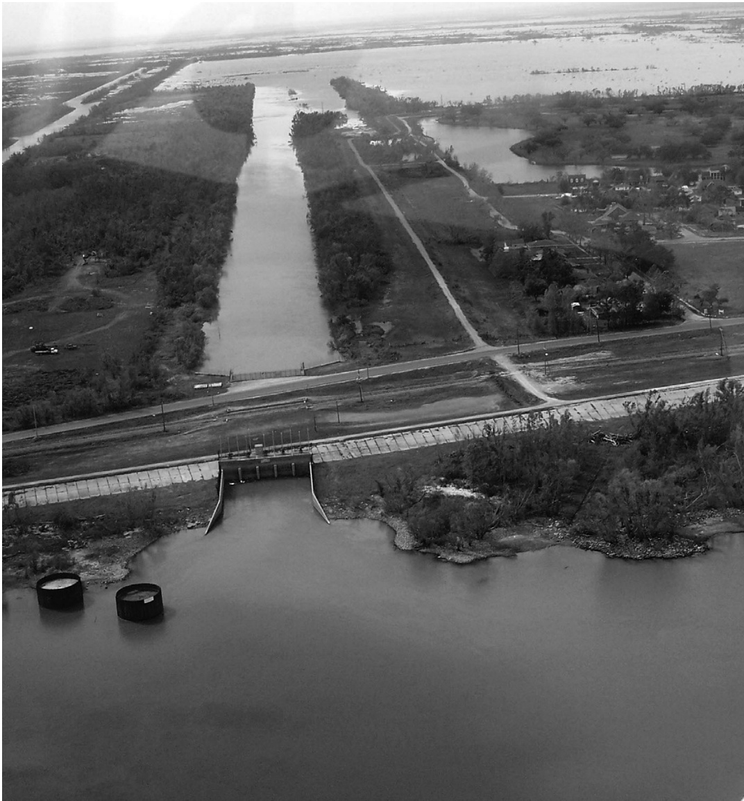
FIGURE 13.10 The Caernarvon Diversion structure on the Mississippi River allows floodwaters to pass through an artificial levee and enter the wetlands of Breton Sound in the distance. (Courtesy J. Day.) (See also color plate.)
