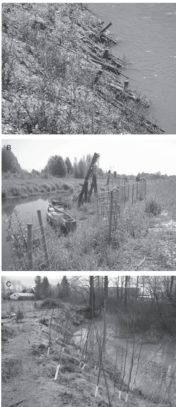
Figure 5.5 Photos of (A) willow stakes to stabilize newly contoured bank following removal of bank armoring (Drau River, Austria) and (B, C) live plantings to restore riparian trees (Fraser River Valley, British Columbia, Canada). Note use of fencing to protect plantings from herbivores. Photos (B) and (C) M. Pearsons.
