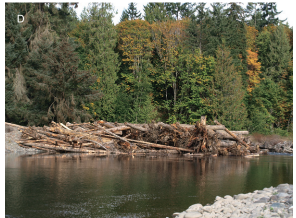
Plate 11 (Figure 5.7) Common instream habitat improvement techniques including (A) placing LWD in a small stream (photo M. Pearsons); (B) boulder weir on an Erriff River, Ireland (photo Dan Kircheis); (C) gravel and wood placement below a Howard Hansen Dam, Green River, Washington State, USA (photo Scott Pozarycki); and (D) engineered logjam Elwha River, Washington (photo M. McHenry).
