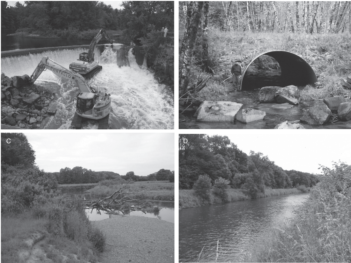
Figure 5.1 Common approaches for restoring longitudinal and lateral connectivity including: (A) dam removal (Souhegan River, New Hampshire; from Pearson et al. 2011, reproduced by permission of American Geophysical Union, Copyright 2011 AGU); (B) a recently replaced culvert with a natural stream bottom (West Fork of Smith River tributary, Oregon, USA); (C) a restored (removal of bank protection) and (D) adjacent unrestored reaches of the River Aggar, Germany. (See Colour Plate 7)
