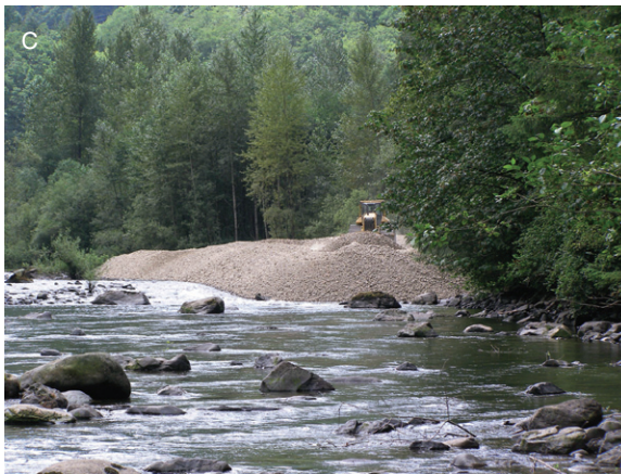
Plate 11 (Figure 5.7) Common instream habitat improvement techniques including (A) placing LWD in a small stream (photo M. Pearsons); (B) boulder weir on an Erriff River, Ireland (photo Dan Kircheis); (C) gravel and wood placement below a Howard Hansen Dam, Green River, Washington State, USA (photo Scott Pozarycki); and (D) engineered logjam Elwha River, Washington (photo M. McHenry).
