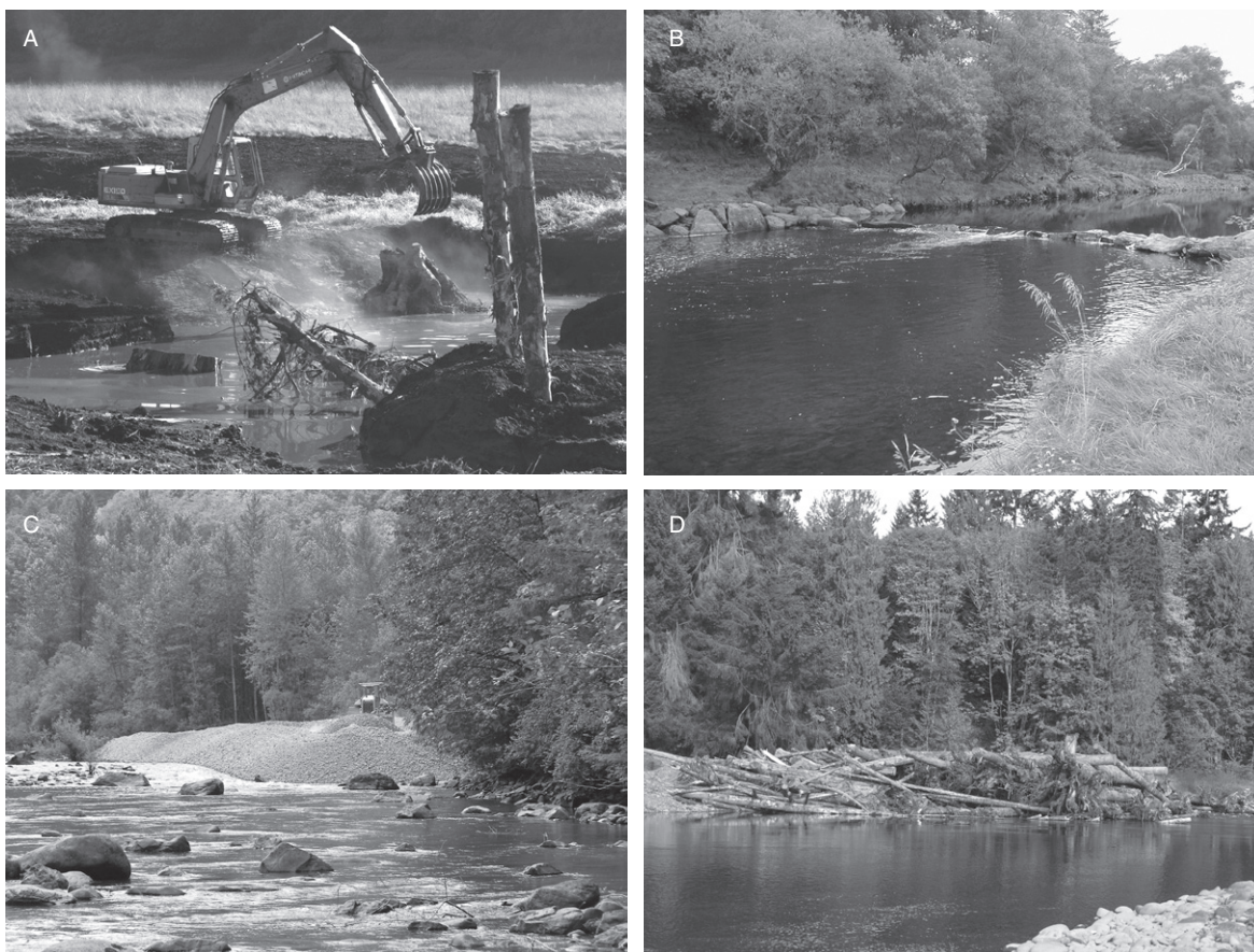
Figure 5.7 Common instream habitat improvement techniques including (A) placing LWD in a small stream (photo M. Pearsons); (B) boulder weir on an Erriff River, Ireland (photo Dan Kircheis); (C) gravel and wood placement below a Howard Hansen Dam, Green River, Washington State, USA (photo Scott Pozarycki); and (D) engineered logjam Elwha River, Washington (photo M. McHenry). (See Colour Plate 11)
