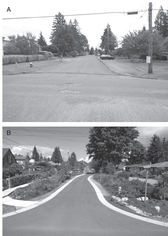
Figure 5.4 Example of (A) before and (B) after narrowing a paved residential street to reduce impervious surface area and creation of bioswales for water retention. Runoff was reduced by more than 90% following reduction of impervious surface and addition of bioswales and vegetation (photos courtesy of City of Seattle Public Utilities).
