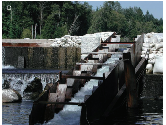
Plate 8 (Figure 5.2) Common types of structures used to pass fish at weirs and dams including: (A) a fish ramp Vara River, Italy (photo Enrico Pini-Prato); (B) a bypass channel for both fish passage and kayaking on Gave de Pau River, France (photo Enrico Pini-Prato); (C) pool and weir type pass at Lower Granite Dam, Snake River, Washington State, USA; and (D) a Denil steep pass at Bennett Dam, North Santiam River, Oregon (photo Ed Meyer).
