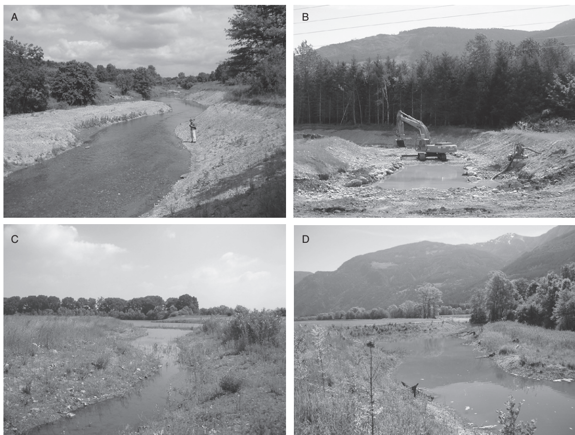
Figure 5.8 Example of (A) remeandering of a formerly channelized stream (River Duhn, Germany); (B) construction of a groundwater channel to create spawning and rearing habitat, Skagit River, Washington State, USA (photo Sarah Morley); (C) reclaimed gravel pit (Rhine River, Germany); and (D) reconnected and reconstructed side channel (River Drau, Austria).
