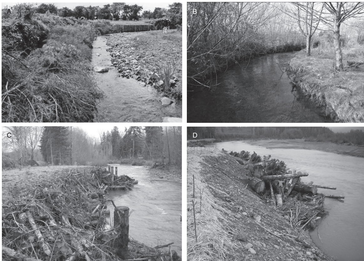
Figure 5.9 Examples of bioengineering approaches for bank protection using brush or logs. (A) Christmas tree revetments to help limit erosion while riparian zone recovers following fencing to exclude livestock on an Irish river immediately after placement and (B) 17 years later (photos Martin O’Grady, Inland Fisheries Ireland). (C, D) Bioengineering bank revetments using large woody debris (photos Herrera Inc.).
