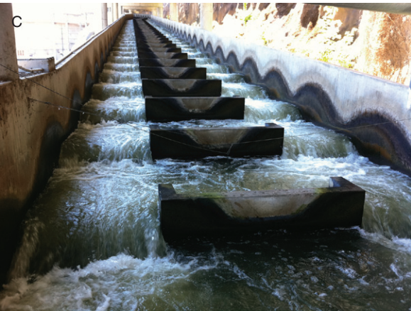
Plate 8 (Figure 5.2) Common types of structures used to pass fish at weirs and dams including: (A) a fish ramp Vara River, Italy (photo Enrico Pini-Prato); (B) a bypass channel for both fish passage and kayaking on Gave de Pau River, France (photo Enrico Pini-Prato); (C) pool and weir type pass at Lower Granite Dam, Snake River, Washington State, USA; and (D) a Denil steep pass at Bennett Dam, North Santiam River, Oregon (photo Ed Meyer).
