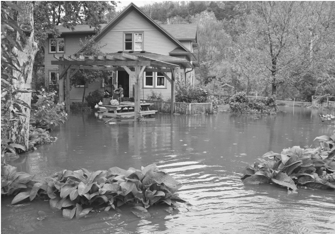
Figure 8.8 Calm waters within the permeable flood fence prevented damage from more forceful flows and debris in the zone adjacent to the Blairs' house during the 2010 flood. (Photo by Bruce B. Blair.)
