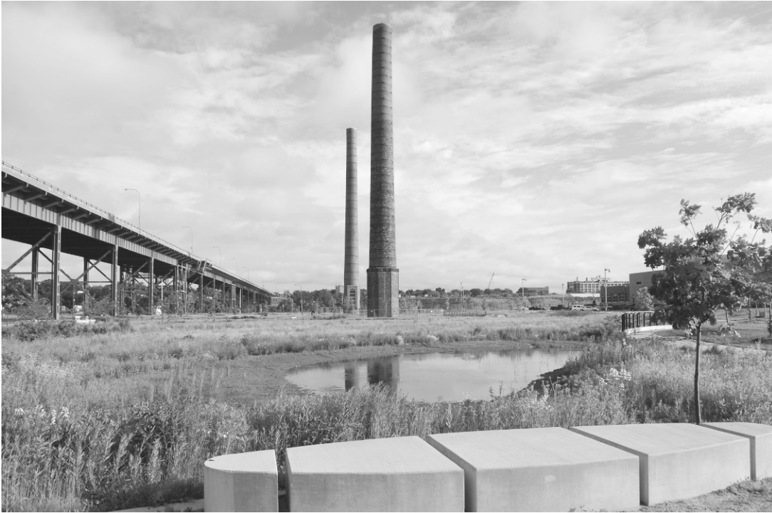
Figure 6.14 A filtration basin planted with native species in Menomonee Valley Community Park, Milwaukee captures and treats runoff from an adjacent light industrial development. Smokestacks are a reminder of the Menomonee Valley's heavy industrial past. (Photo courtesy of Wenk Associates.)
